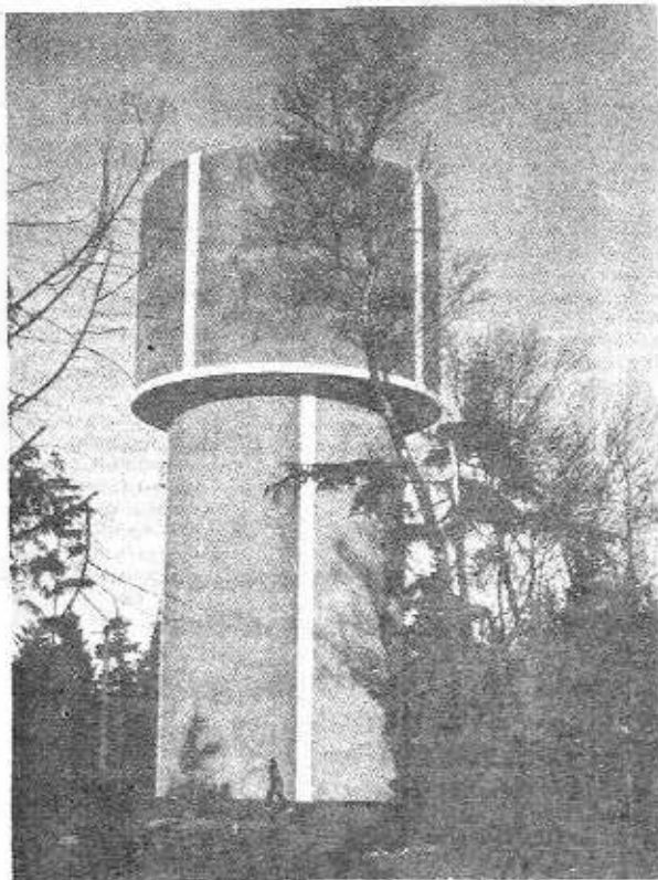
356,000 Imp. Gal. Water Storage Tower, Municipality of Delta, B.C. designed by Faliszewski Engineering Ltd.
