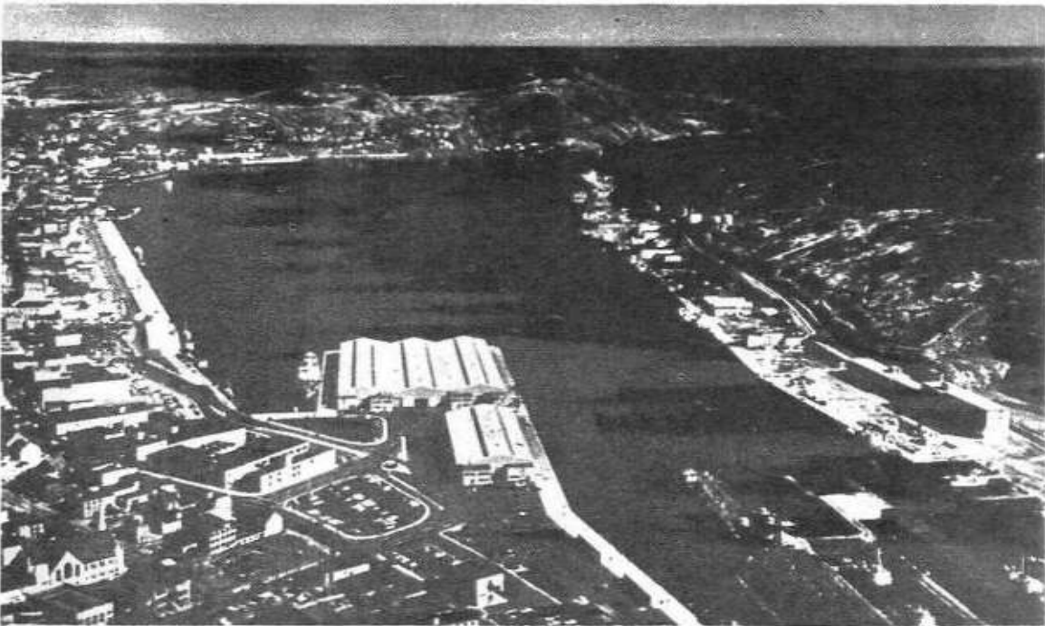
Harbour in St. John's, Newfoundland, built by the Foundation of Canada Engineering Corp. Ltd., under the supervision of J.M. Chmieleński.
